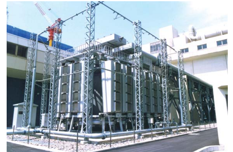
Generator step up transformer 1,450MVA, 26.325/525kV
