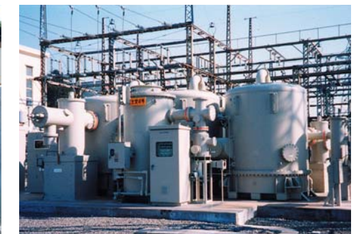
SF 6 gas insulated transformer 100MVA, 154/66/10.75kV
