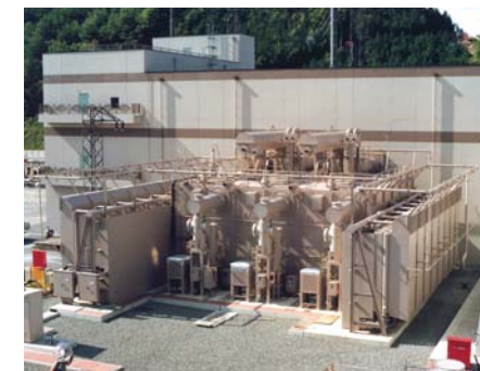
Converter transformer (HVDC) 872MVA, 500/110/110kV
