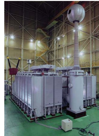
Experimental UHV transformers \frac{3000}{3} / \frac{3000}{3} / \frac{1200}{3} MVA, \frac{1050}{\sqrt{3}} / \frac{525}{\sqrt{3}} / 147 kV
