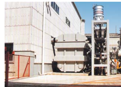
Short-circuit transformer connected to the short-circuit generator inside the laboratory. Voltage: 14.4/12.6–12.6kV (60Hz) 12.0/10.5–10.5kV (50Hz) Frequency: 50/60Hz Capacity: 216MVA
